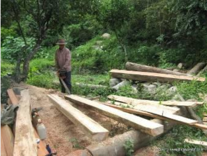
Cutting the posts
