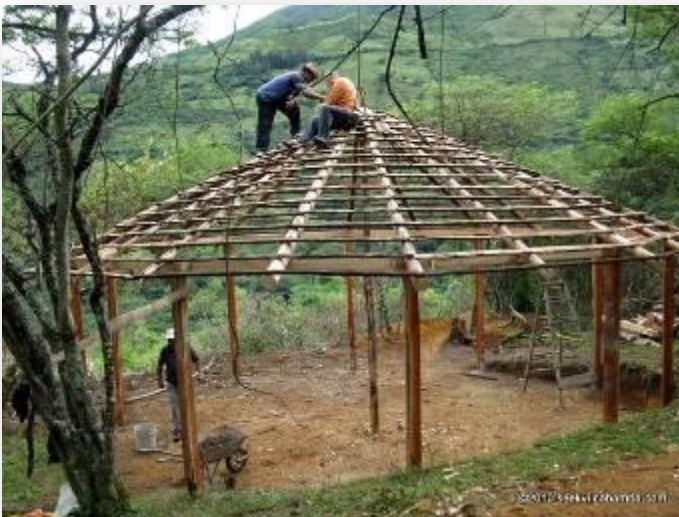
Preparing the roof for the straw
